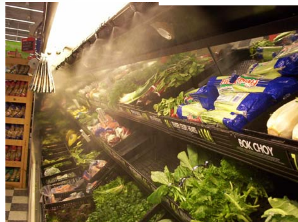
UltraMist provides the finest mist and 100% coverage in any style case.
