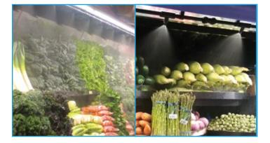
Corrigan engineers the activated oxygen ( $O_3$ ) to sanitize the mist bar, nozzles and drain lines. The precise amount of  $O_3$  is metered for the correct duration to effectively sanitize the system. Typically, it is programmed for just two minutes in the middle of the night or early morning hours. TriOBreeze is residue-free and does not require expensive chemical solution refills.
